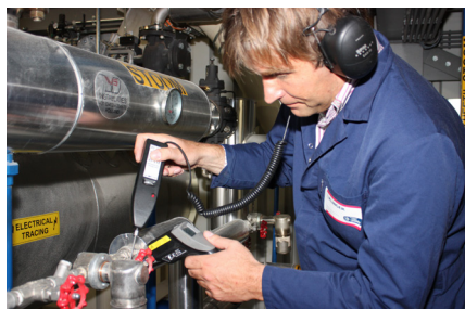
An experienced KLINGER steam technician thoroughly checking the overall performance of an inverted bucket by using ultrasonic and thermal equipment.
