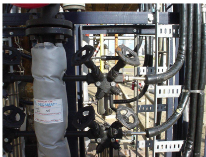
An Armstrong steam trap, made of polished stainless steel, mounted on a condensate collection steam manifold. The insulation blanket ensures reduction of the heat and energy losses.
