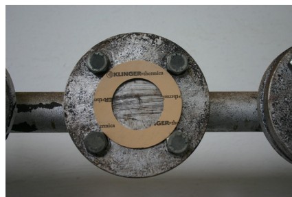
A KLINGER®thermica seal on one of the flanges of the boiler house of our own company
