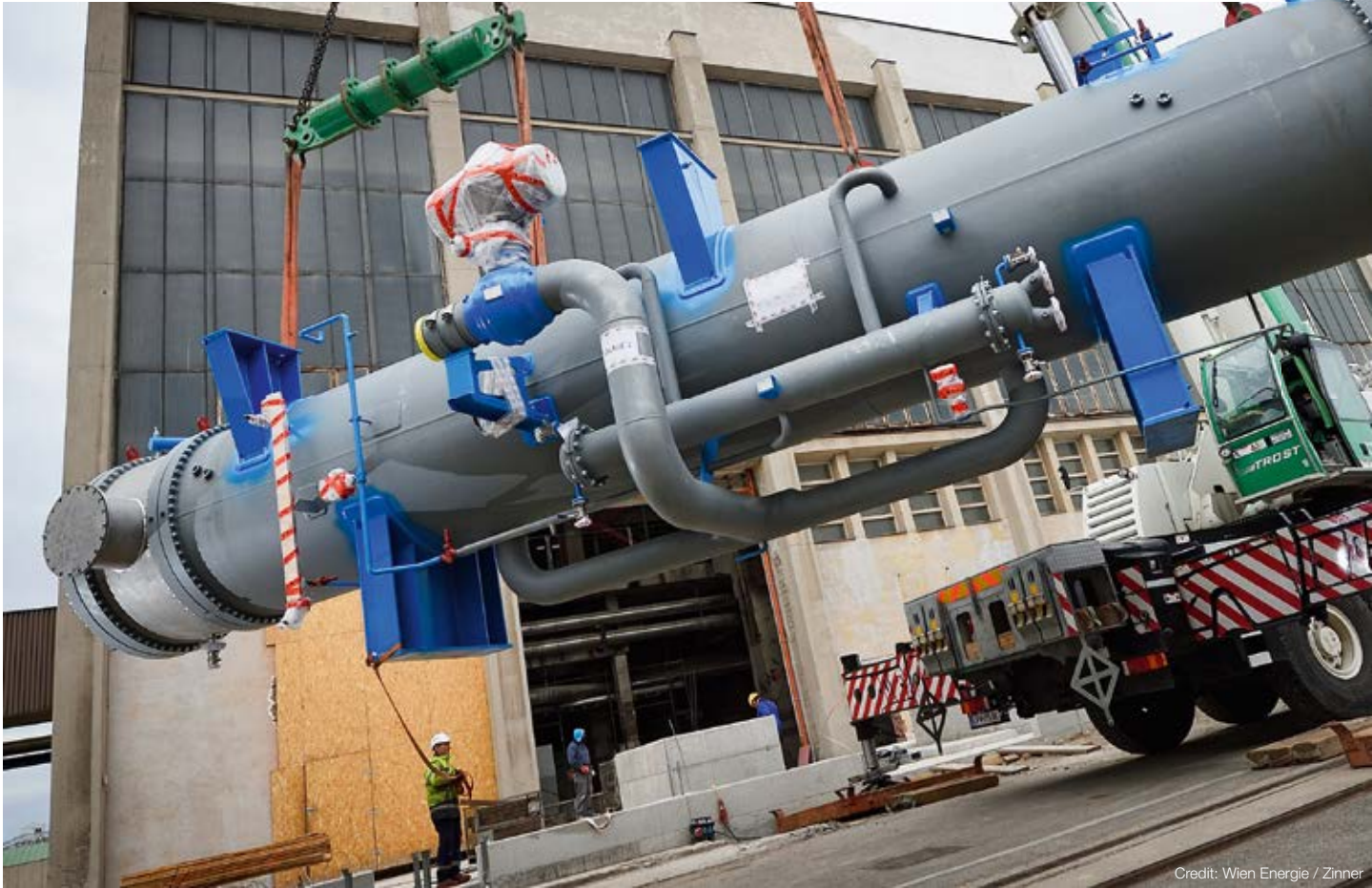
One of several KLINGER Ballostar KHSVI ball valves, from DN 250 up to DN 400, installed on the heat pump
