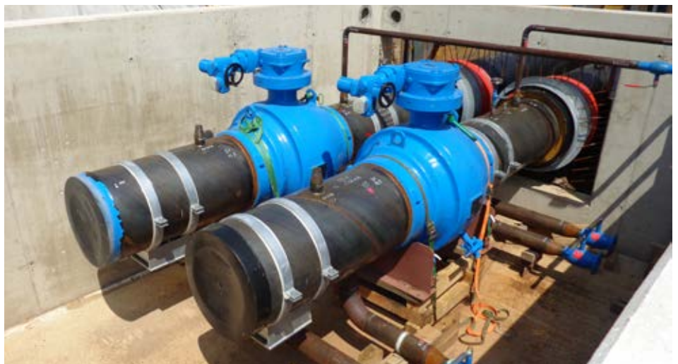
Two Klinger Ballostar® KHSVI VWS DN 700 were installed in July 2016
