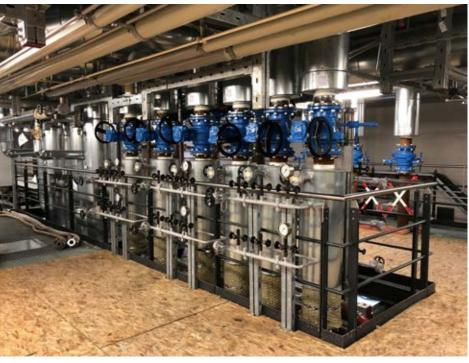
Due to their design, butterfly valves are especially prone to the effects of scaling
